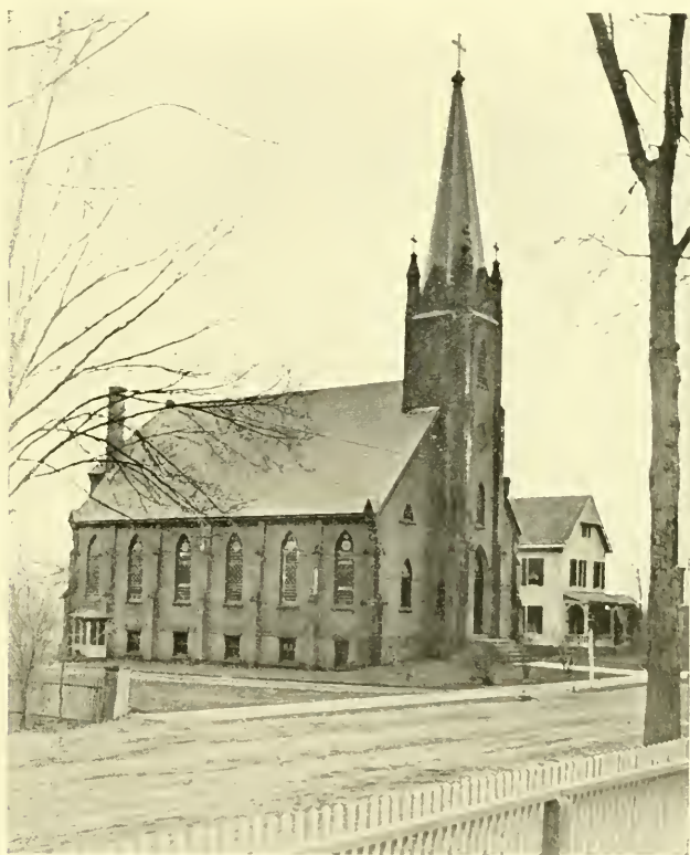
CATHOLIC CHURCH, HAMDEN, CONN.
